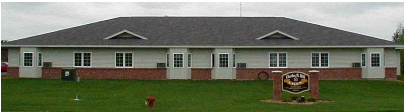
Charles Hill Villa, owned and managed by Impact Seven, is home to low-income elderly residents in Park Falls, Wisconsin. It is one of a number of projects that Impact Seven has partnered with Johnson Bank to complete.
