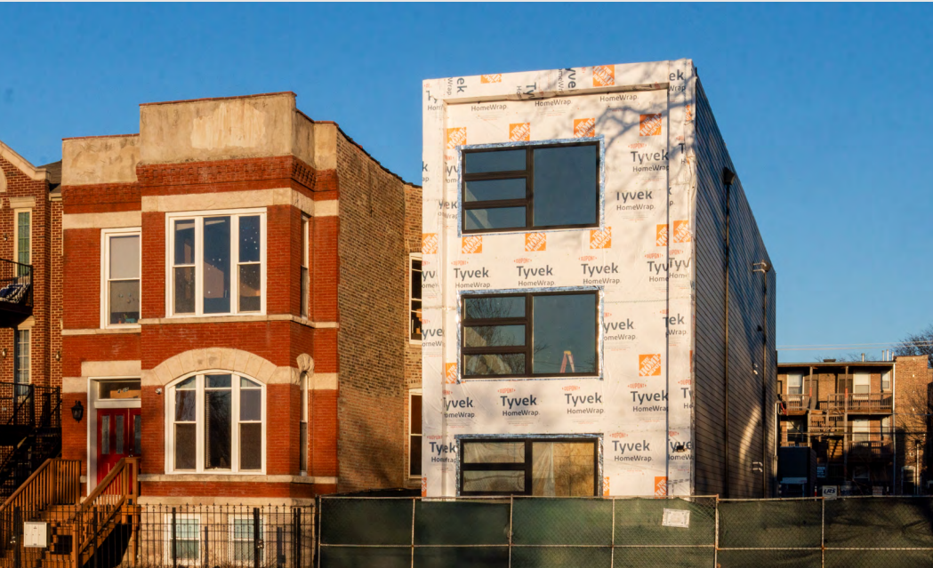
CoVantage Credit Union leveraged FHLBank Chicago's Community Advance in 2025. Construction of three multifamily units in Chicago's Bronzeville neighborhood is underway, expanding housing supply in Illinois.
